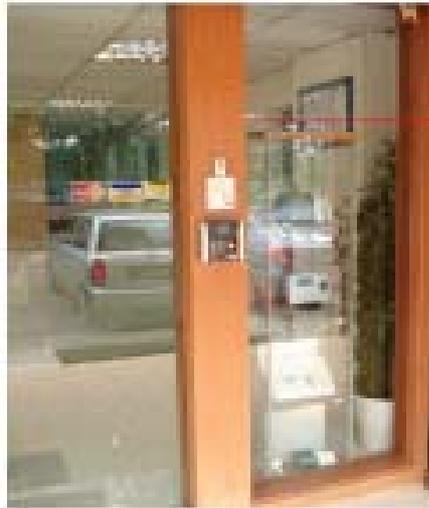
The wooden panel is constructed at the side of the glass door to mount FingerTec® reader on the wooden panel. The connection wires shall be hidden in the wooden panel.
