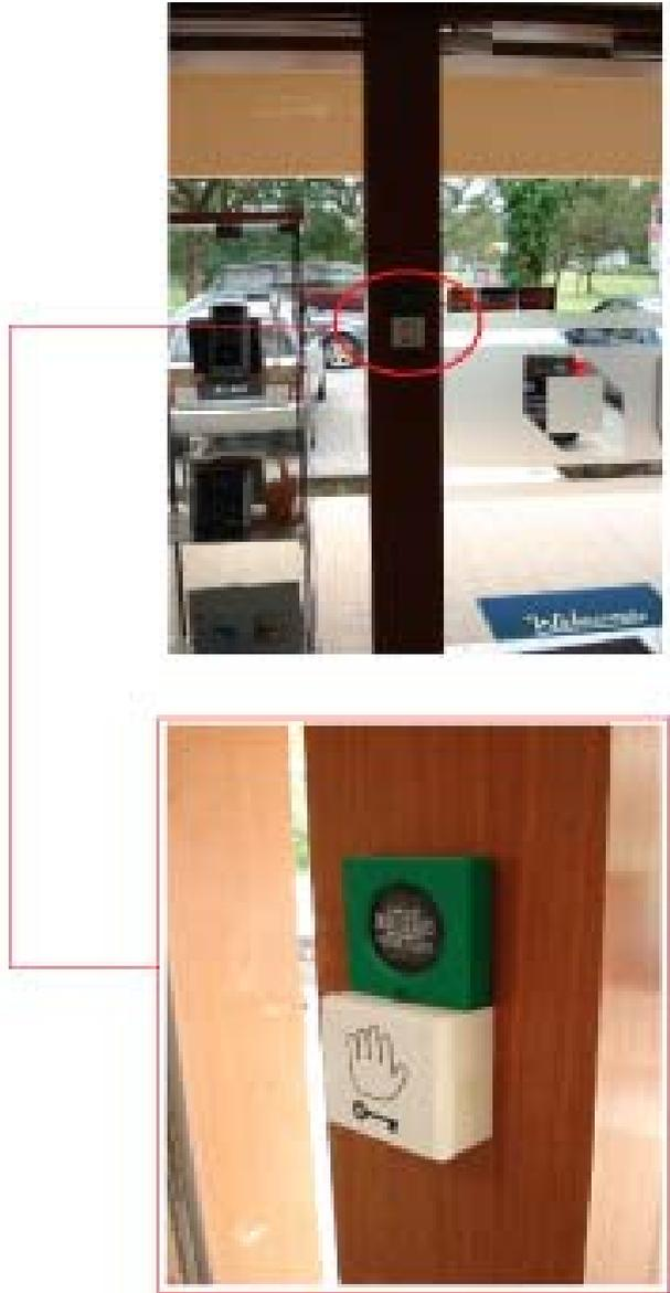
The accessories shall be mounted on the wooden frame properly with connection wires hidden in the wooden panel.
