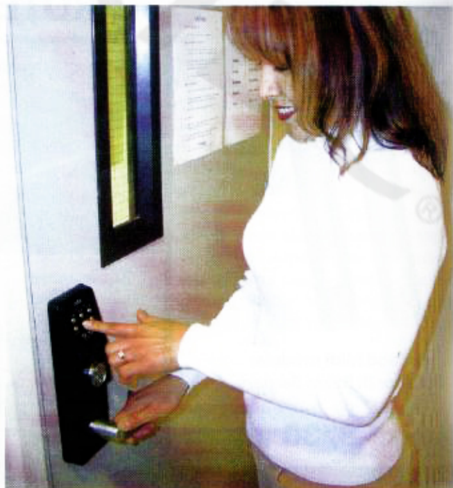
Stand-alone computer-managed locks provide an audit trail of 1,000 events.
